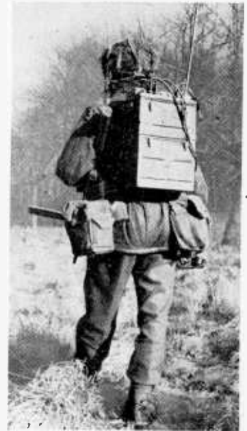
FM "WALKIE-TALKIE." This American Signal Corps pack transmitter-receiver, type SCR 300, has been used to some extent by the British Army. The set, measuring 17 x 12 x 7 in., weighs 35 lb.
